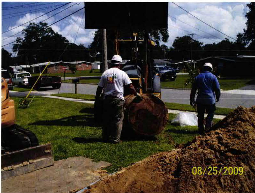
Picture 2: UST 1227Dove.
